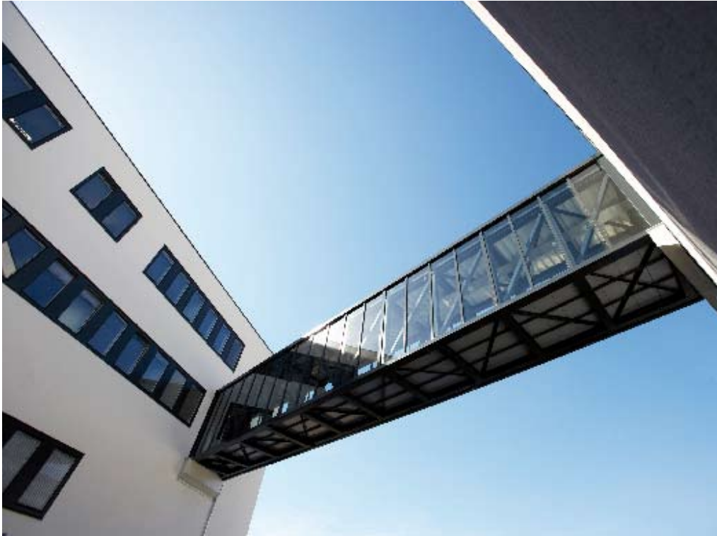
The new Impulse Centre for Materials (IZW) with connecting gallery.
