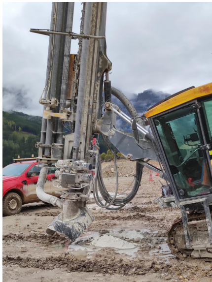
Fig 2: Sensor on drill rig
